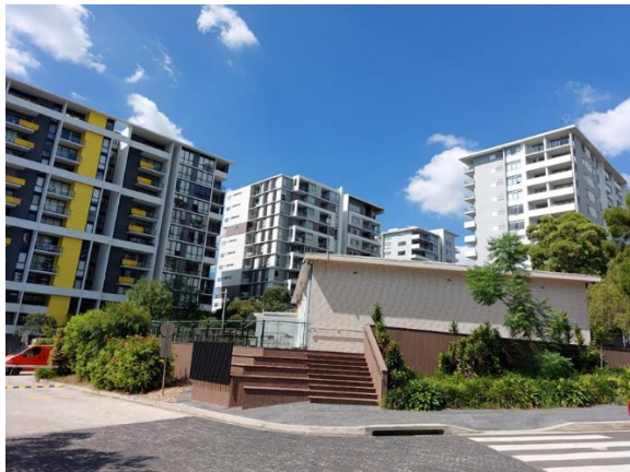
Figure 14 - View north of the rear of the admin building
