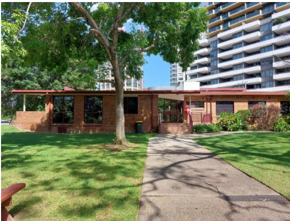
Figure 19 - East view of the administration building (to be demolished)
