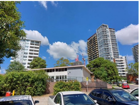
Figure 13 - View east of the rear of the admin buildings
