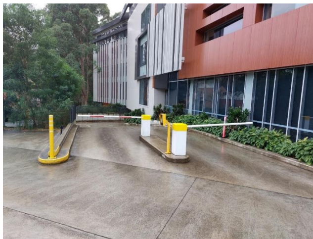
Figure 34 – Ramp to the MALC building car park.
